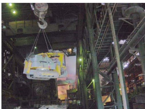
The Brokk 180 is lifted into the plant.
