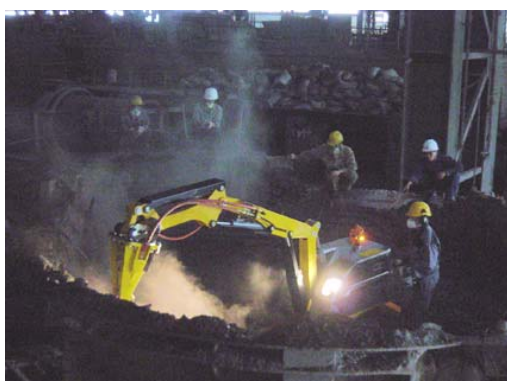
Brokk 180 with breaker, cleaning the EAF.
