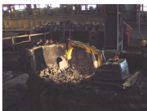
Brokk with bucket clears out the debris.
