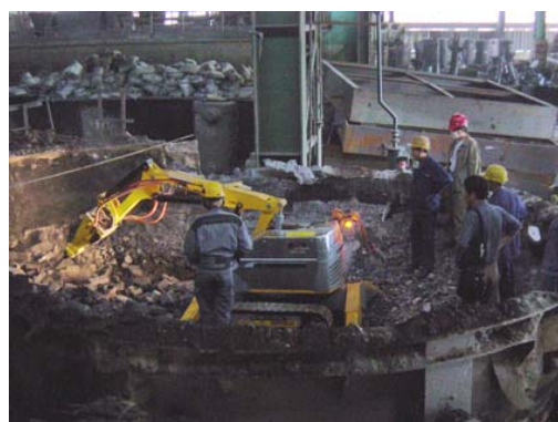
The operator has a good view of the work.
