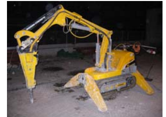
Night time shift, Brokk 90 with hydraulic breaker
